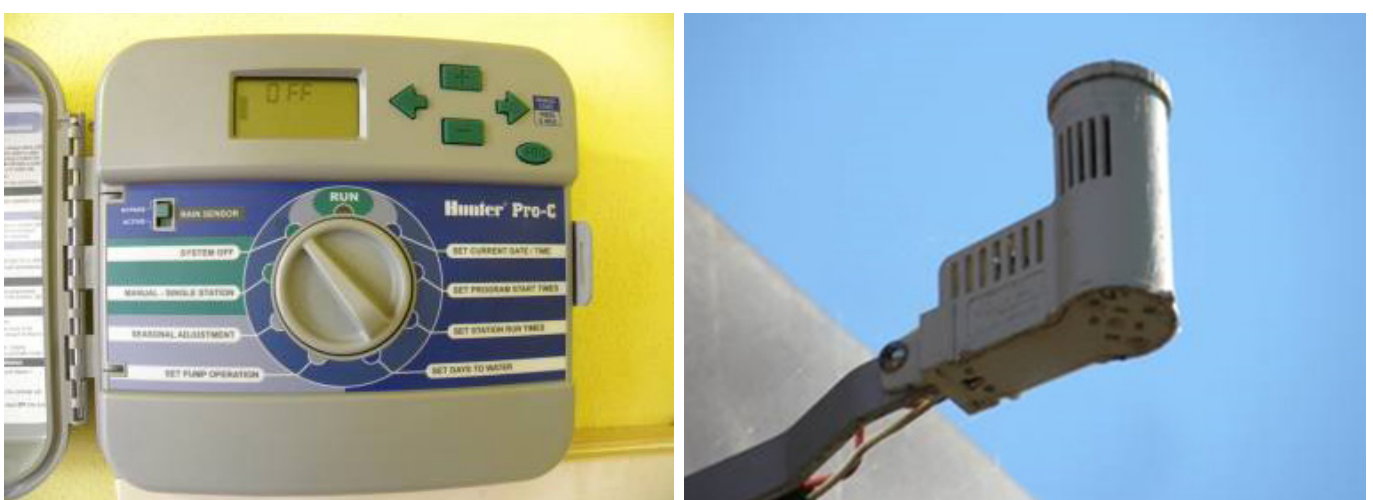
Figure 4 Control unit, rain sensor Source: own photograph on site
