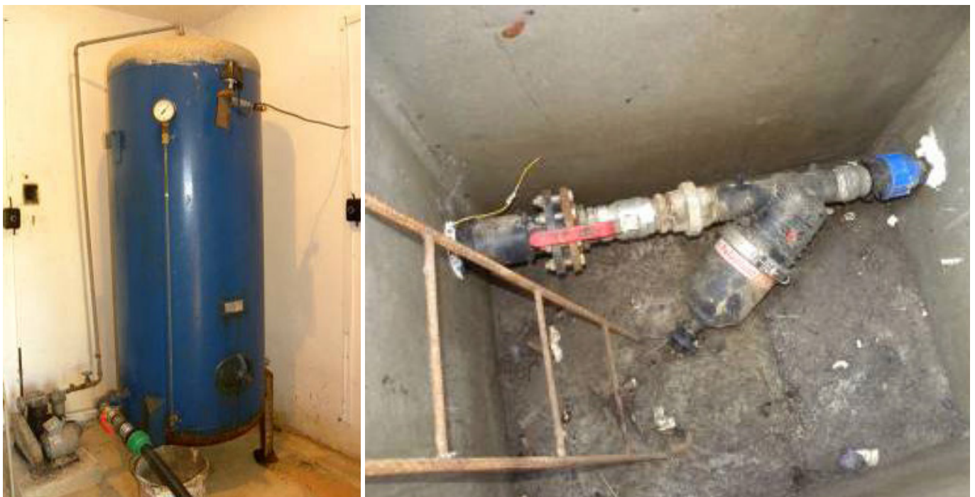
Figure 2 Pressure tank, control shaft
